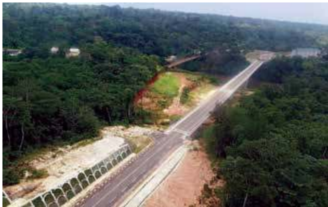
Central-West Africa interconnection, bridge over the Cross River between Cameroon and Nigeria
