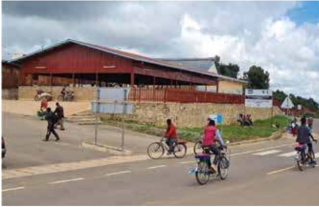
A women's market in Ethiopia constructed as part of the Bank-funded Base-Rukomo Project
