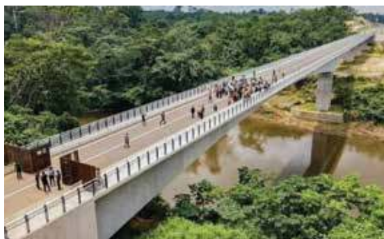
Bridge connecting Cameroon and Congo as part of the Ketta-Djoum Road
