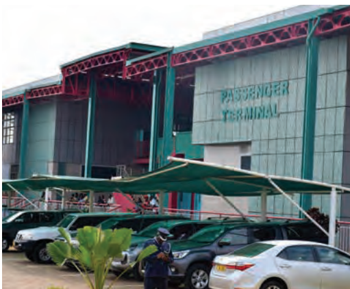
One Stop Border Post on the Nacala Road Corridor between Malawi and Zambia
