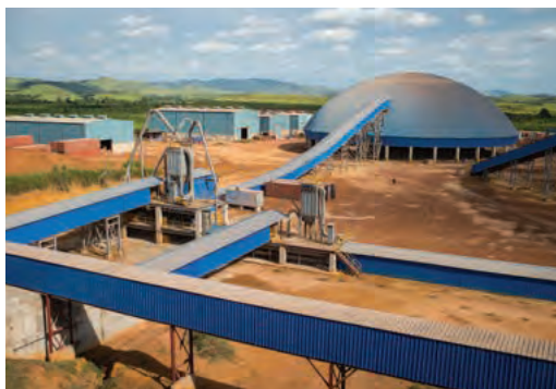
Nyumba Ya Akiba Cement Plant Project, Democratic Republic of the Congo
