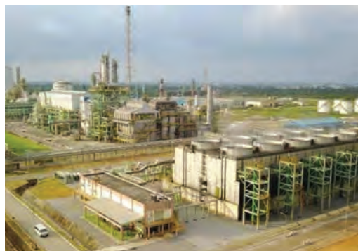
The Nigeria Indorama Fertilizer Plant Project supports the country's agricultural sector, which accounts for 25 percent of its GDP.
